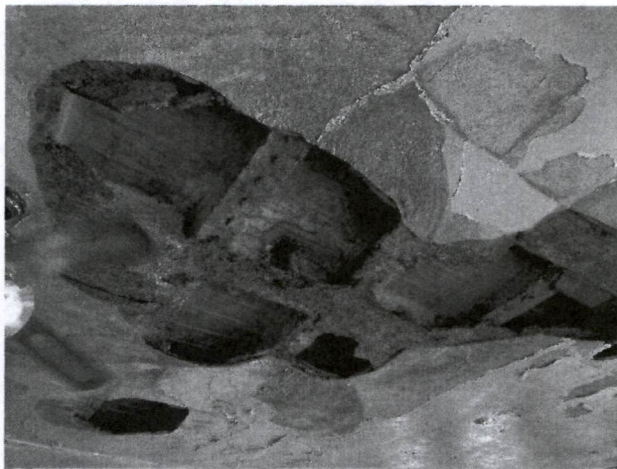
Left: Close up view of damaged plaster ceiling and concrete roof deck. Right: View of central beam with differing roof structures at either side.
