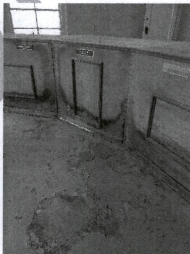
Left: Close up of original paint layers behind spalled contemporary layers. Center: View of water damage at Dias and concrete floor. Right: Close up of paint layers at concrete floor.
