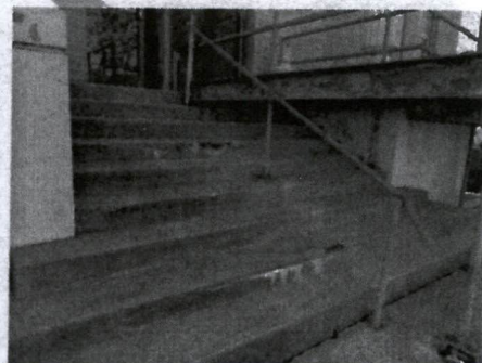
Left: Peeling paint and cracking at the northeast cheek wall. Center: Northeast planter with significant cracking. Right: View of cracked and spalling concrete at the north steps with white efflorescence.
