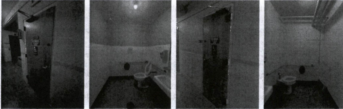
Basement Accessible Men's and Women's Restroom
