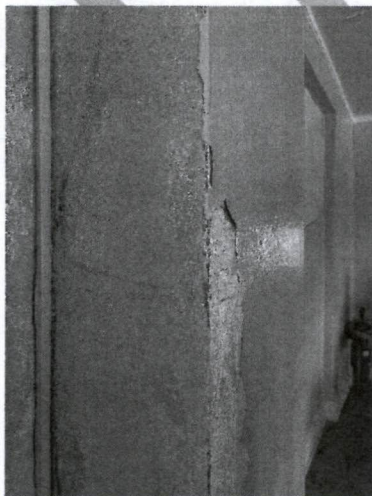
Left: Close up of original paint layers behind spalled contemporary layers. Center: View of water damage at Dias and concrete floor. Right: Close up of paint layers at concrete floor.
