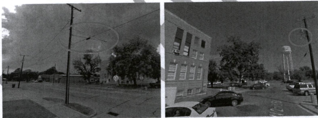
Left: Example of streetlighting on W. Dallas Avenue. Right: Example of streetlight at NW. Second Street.
