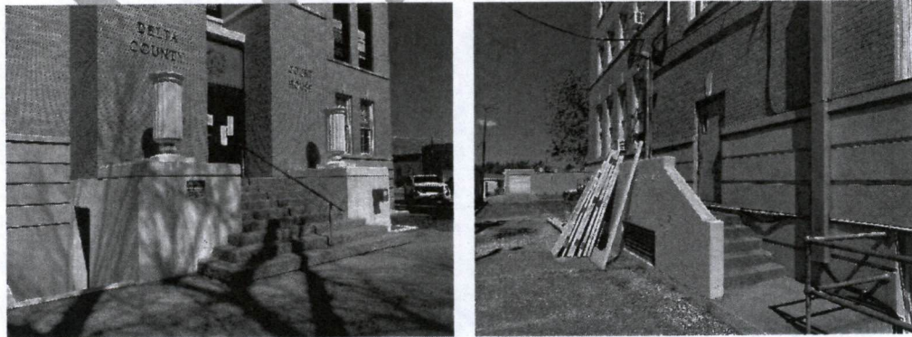
Left: South Entry Porch. Right: West Entrance.
