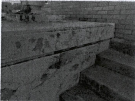
Left: Peeling paint and cracking at the northeast cheek wall. Center: Northeast planter with significant cracking. Right: View of cracked and spalling concrete at the north steps with white efflorescence.
